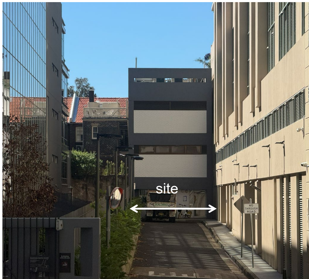
existing southern elevation – Jenkins Street
