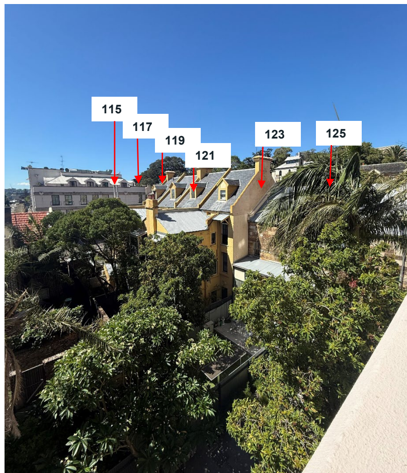
rear view of terraces to the north of subject site on Kent Street
