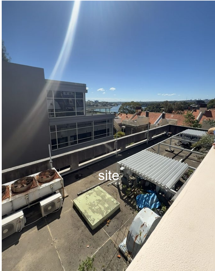
view north-west of existing roof from Level 6 Highgate Apartment
